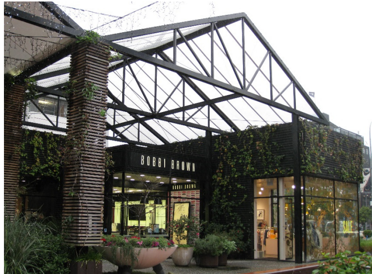
Figure 13: The clear PVC roofing on the two side canopies works well in letting in maximum light to the circulation spaces (especially in the winter).
