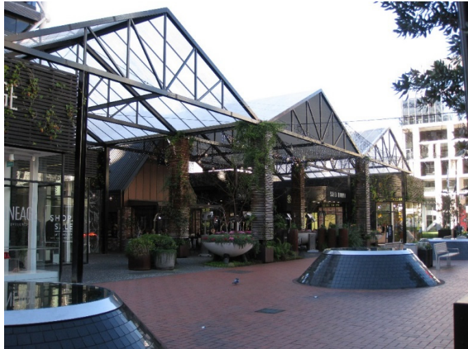
Figure 11: A winter view from the Te Ara Tahuu pedestrian walkway illustrates the three gable canopies with different roofing.
