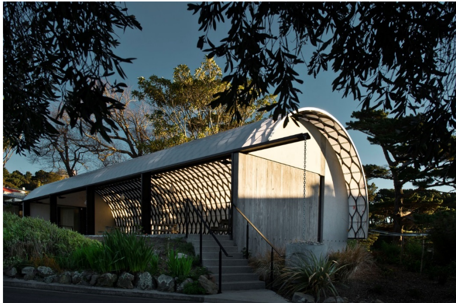
Figure 37: The afternoon sun is filtering through trees to pattern the membrane roofing
