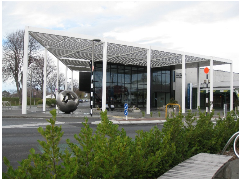
Figure 45: A view of the canopy from across Williams Street showing the waterproof roof leading to the main entrance.
