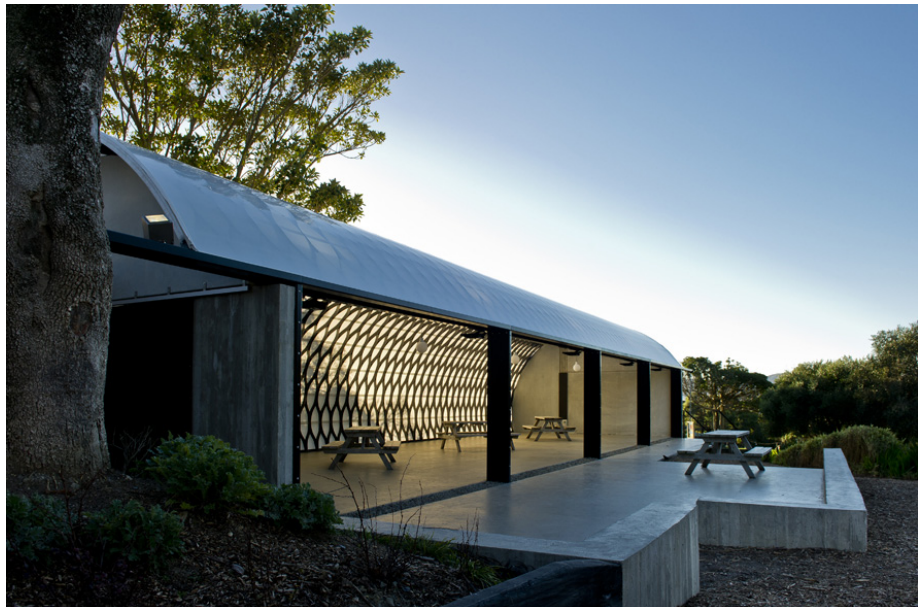
Figure 38: An image the pavilion exterior taken soon after it opened. When the blinds are rolled up the space becomes a large verandah.
