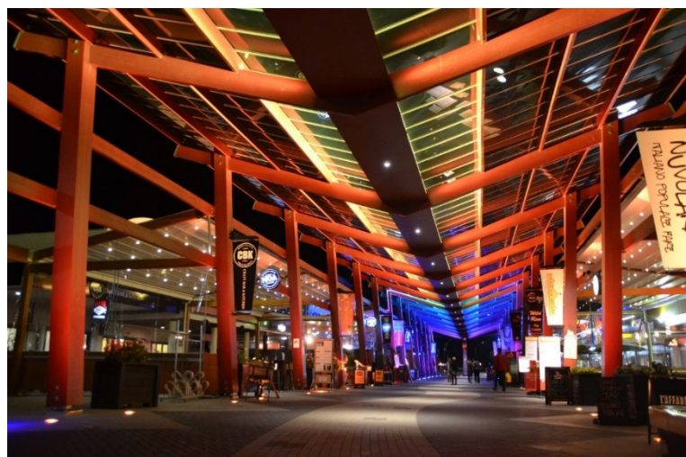
Figure 21: Decorative lighting is used to enhance the canopy in the evening.
