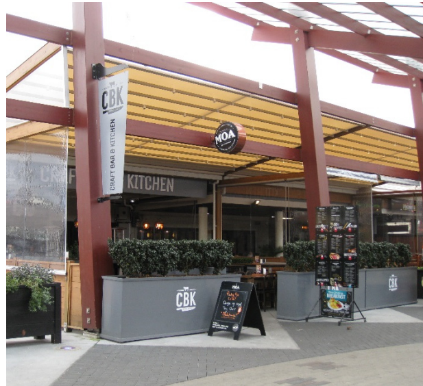
Figure 22: The retractable canopies extend outwards from the front of each restaurant to the central walkway.
